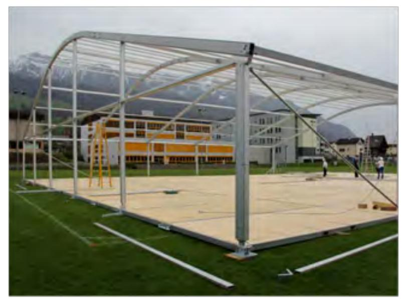
All segments of the heavy burden floor are delivered in the format 2,5x10m as a ready-toinstall component and can be positioned upon all requirements. The complete anchorage of all lifting forces is derived by the
